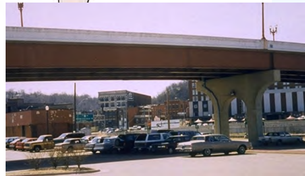
Photo of Existing Overpass
